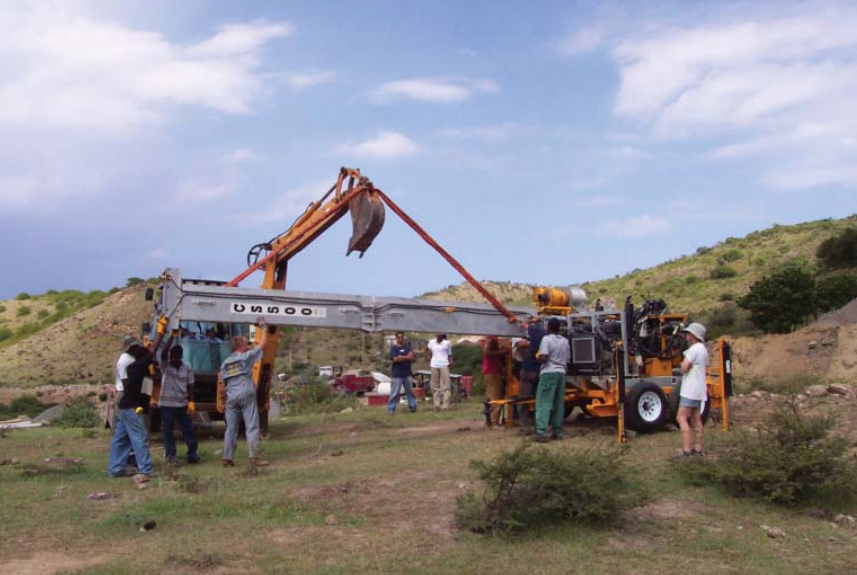
Drilling rig set up, Montserrat (photo by Dennis Nielson)
