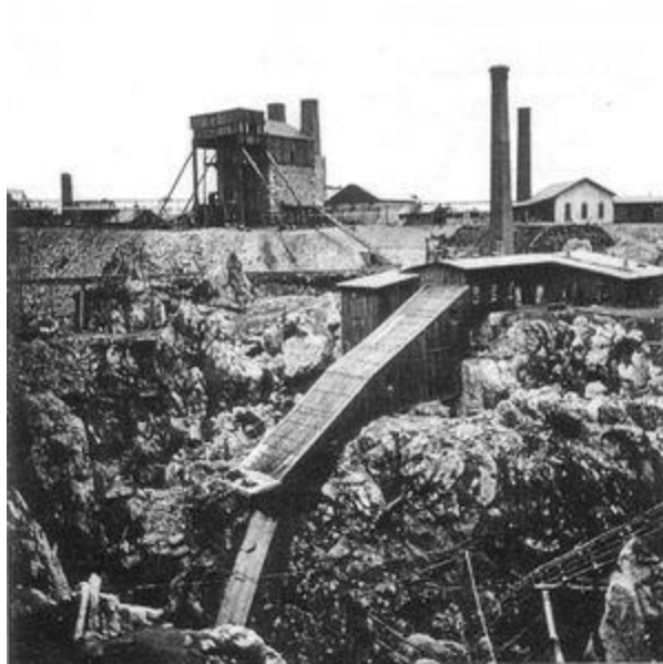
Figure SP.1: Uberroth Mine with “The President” engine house (at the rear) ca. 1876. (Kaas, 2016)
