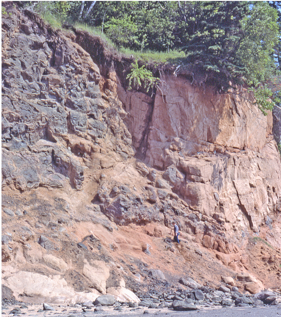
Figure 41: Paleo-talus cone in cross-section at station 9 (Stop 2.2) as it appeared in 1986. On the left is a fault block of North Mountain basalt with a buttress unconformity with younger eolian McCoy Brook Formation on the right, containing a well defined talus cone of basalt cobbles derived from the immediately adjacent paleocliff. Some of the blocks have rolled tens of meters away over the dune surface, while others have moved only slightly away from the cliff.
