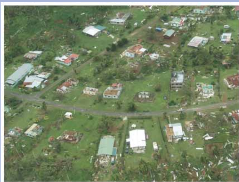
FIG. SB4.2. Widespread damage occurred in the village of Nikaupara on the island of Aitutaki in the Southern Cook Islands caused by Tropical Cyclone Pat in February 2010. (Photo Credit: Mr. Johnny Hosking in liaison with Air Rarotonga)
