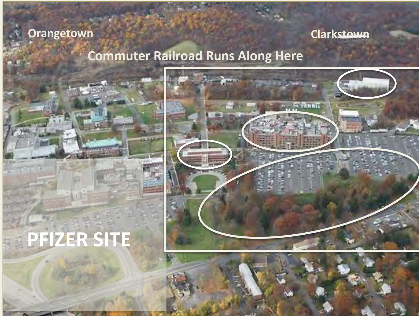
Buildings 140, 100, 170, adjacent parking areas and tree buffer
