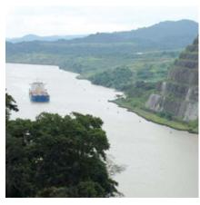
14,000 ships travel the Panama Canal each year. Before the current expansion project, the Culebra Cut (right) was widened in 2001 by 222 meters in some places.
