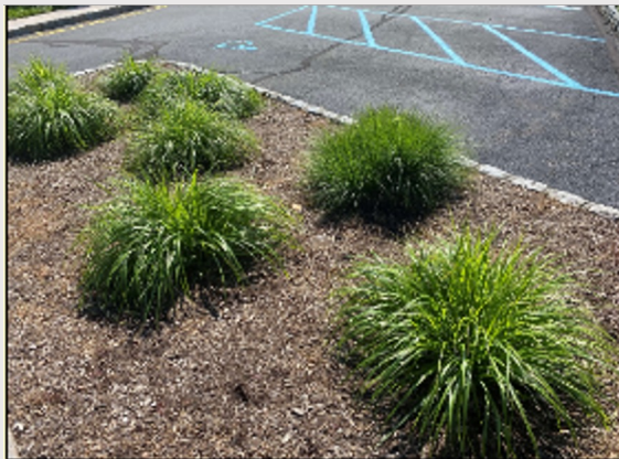
Valley Cottage Library - Vegetated swales
