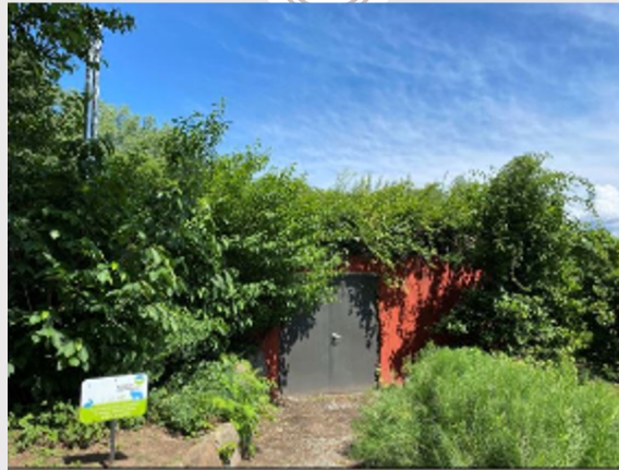
Rockland County Country Club - Green Roof
