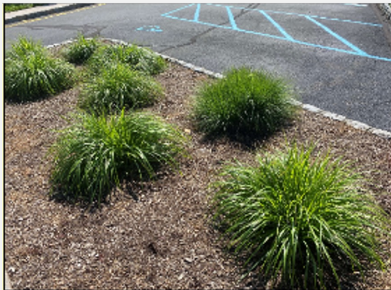
Valley Cottage Library - Vegetated swales
