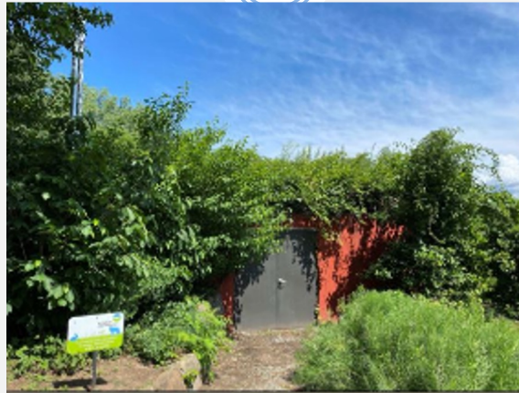
Rockland County Country Club - Green Roof
