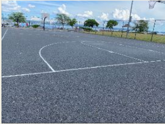
Nyack Memorial Park Permeable pavement
