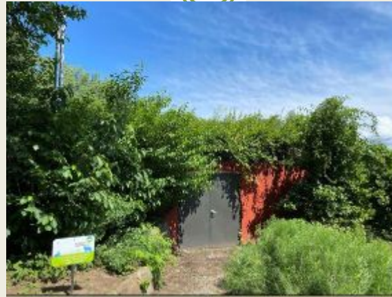
Rockland County Country Club - Green Roof
