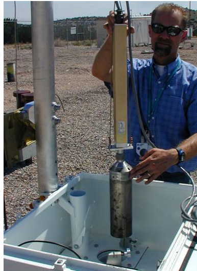
Installation of Integrated Sensor Simulator with DWR in WTU Borehole
