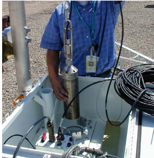
Installation of Sensor Simulator in WTU Borehole
