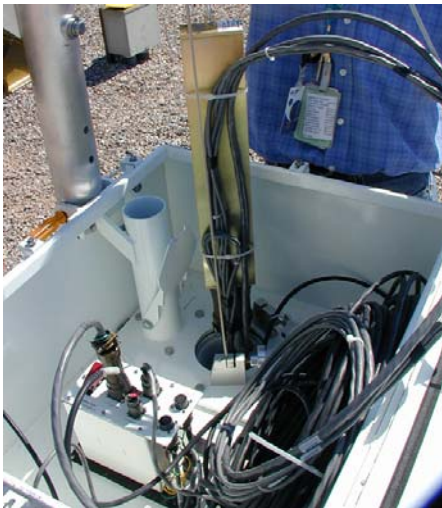
Installation of DWR in WTU Borehole
