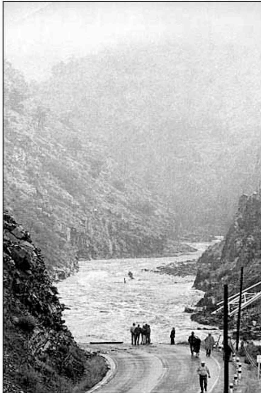
Rescuers stand near a washed-out section of U.S. 34 just west of The Dam Store, looking west into The Narrows of the Big Thompson Canyon following the Big Thompson flood of July 31, 1976. Reporter-Herald file photo
