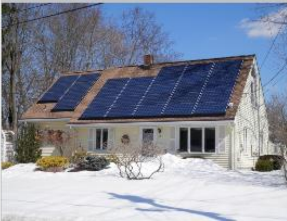
Rooftop in Tappan NY
