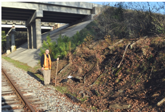
Figure 32b. Bethany Church outcrop is in poor condition in December 2010 showing locations of both bridge footings for US421. The newer eastbound bridge over US421 is in the foreground and the concrete apron has covered important parts of the original outcrop. Photograph taken in December 2010.
