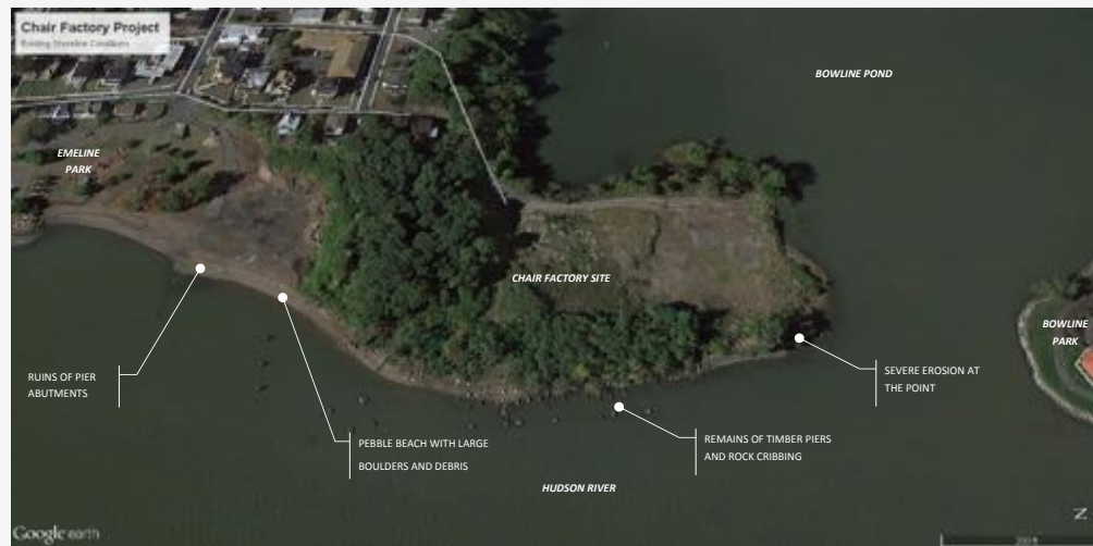
CHAIR FACTORY SITE—EXISTING SHORELINE CONDITIONS
