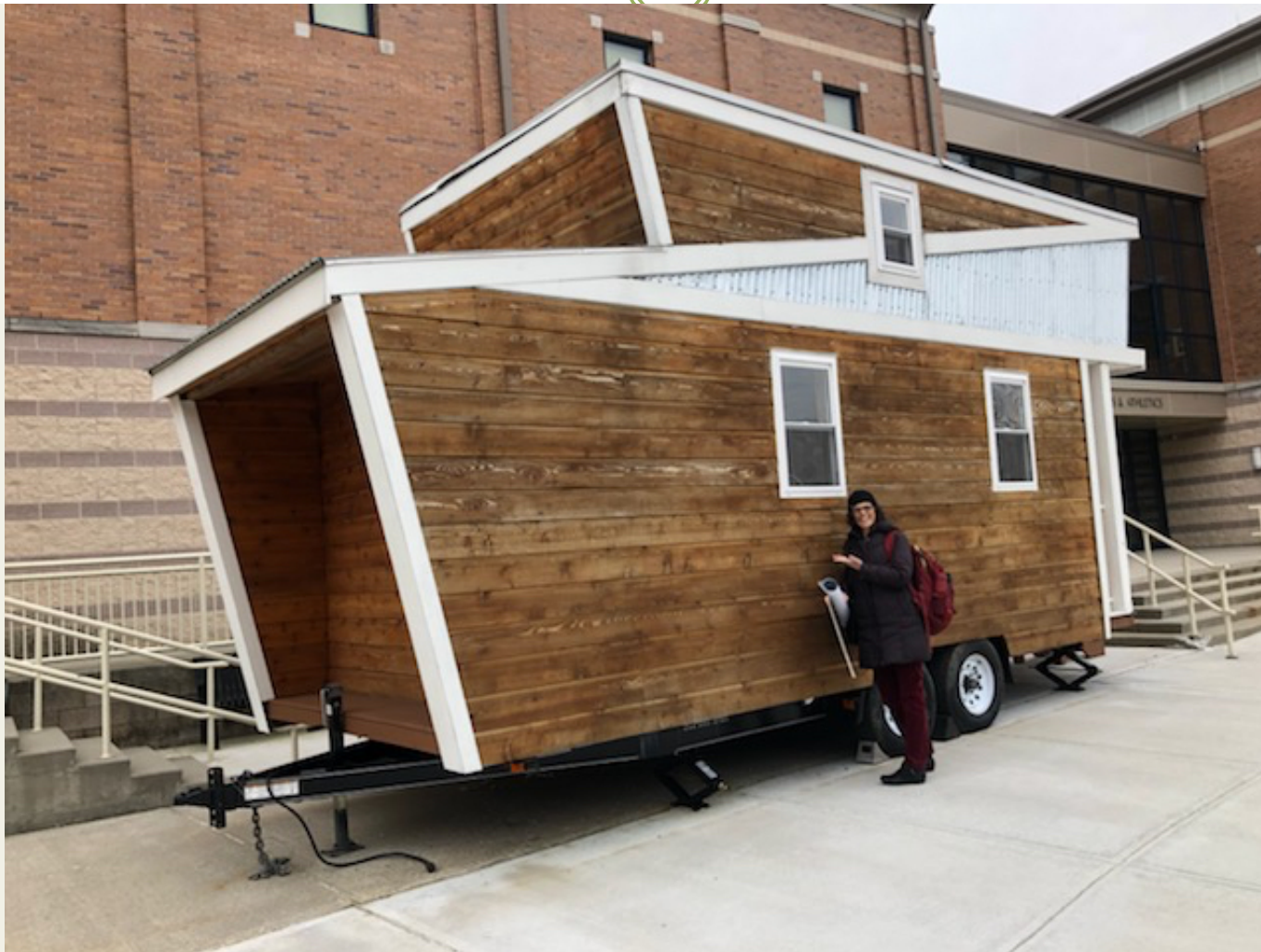
Student Built Tiny Construction at Irvington H.S.
