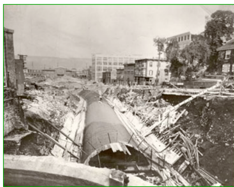
Saw Mill River Being covered – from Saw Mill River Coalition website
