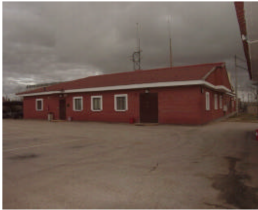
Figure 12. Central Recording Facility at Sonseca
