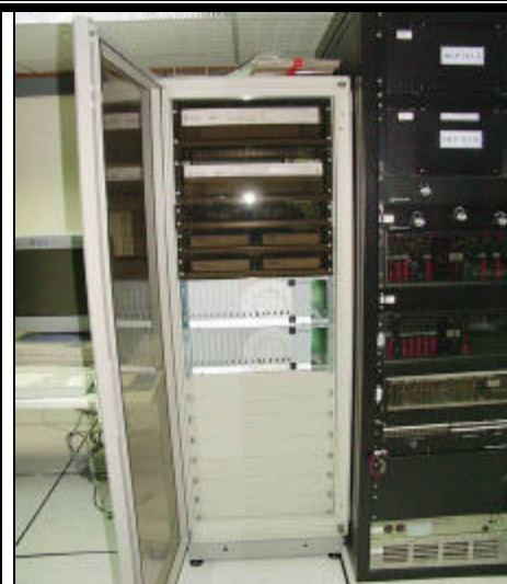
Figure 11. Front of new equipment rack at CRF, primary and back-up DAC on top, two each authenticators below DAC, 4 each RM-4s below authenticators, CRF communications modems below RM-4s. Older AFTAC rack to the right.
