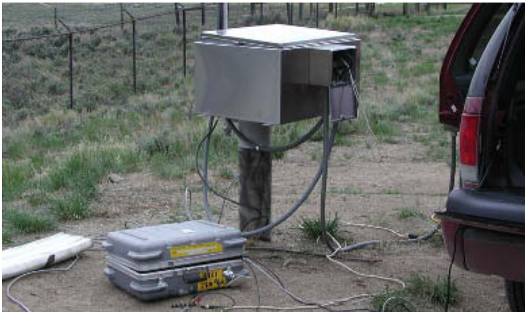
Figure 6. SSS Testing at PSRF
