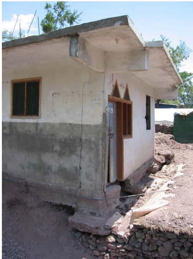
*Sarasha Village: one of the few houses that did not collapse along the strip of destruction. Note fractures widening downward. It appears that this building was damaged by deformation of the foundation, not by shaking.*
