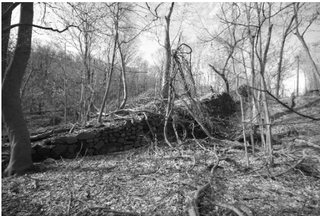
Ramp of the Gravity Railbed, Hook Mountain State Park near Landing Road, Congers, New York
