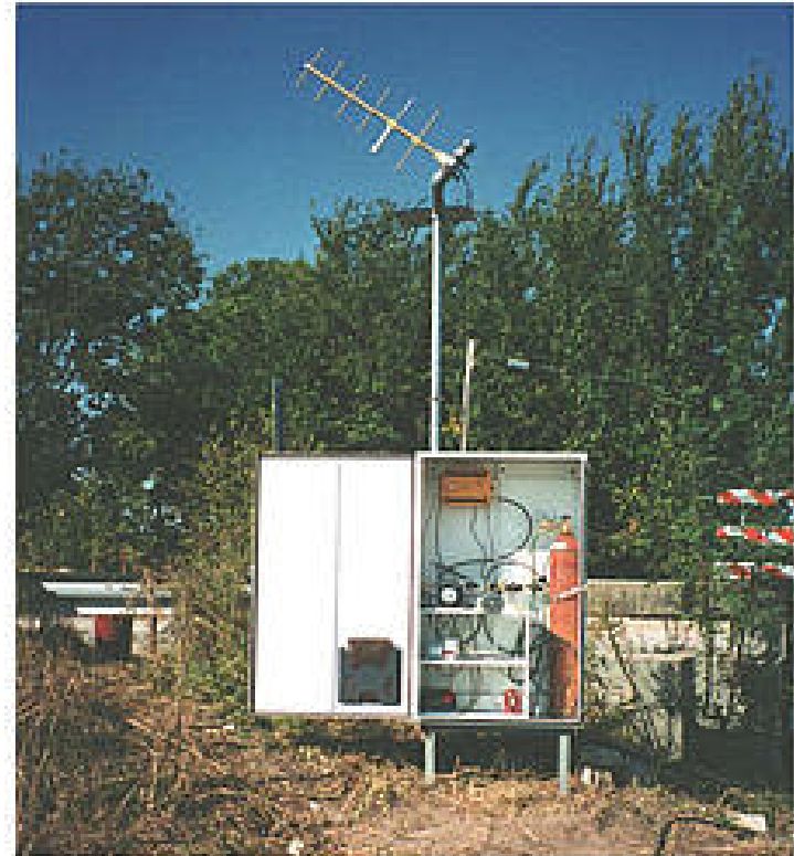
Most USGS stream-gaging stations transmit river stage and other water information directly to geostationary satellites and on to a national hydrologic data network that disseminates information to cooperating agencies and to the public through the Internet.
