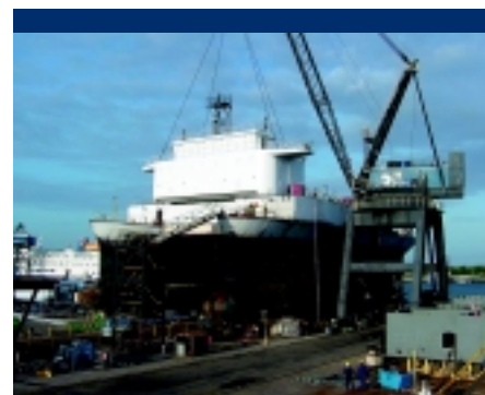
Figure 14. The SWATH ship, R/V Kilo Moana , under construction. This new Ocean Class vessel will join the academic research fleet in 2002. Photo courtesy of R. Hinton.
